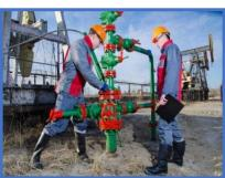
Christmas trees are used on both sub-surface and subsea wells. It is common to identify the type of tree as either "subsea tree" or "sub-surface tree". Each of these classifications has a number of variations. The primary function of a tree is to control the flow, usually oil or gas, out of the well. A tree may also be used to control the injection of gas or water into a non-producing well in order to enhance production rates of oil from other wells.
