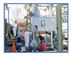
Others are very large with several transformers and dozens of switches and other equipment. Substations generally contain one or more transformers, and have switching, protection and control equipment. In a large substation, circuits breakers are used to interrupt any short-circuit or overload currents that may occur on the network. Smaller distribution stations may use Autoreclosers or even fuses for protection of branch circuits.
