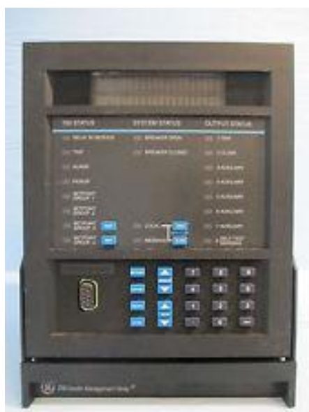
GE Multilin Relay 469 Simulator
