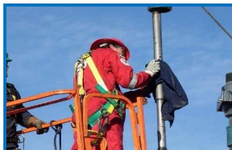
Wireline operations can be done inside the tubing without killing the well, by means of a lubricator connected to the wellhead. Operations can be carried out under pressure and even without stopping production. Further, wireline operations are performed quickly due to the use of lightweight, highly mobile equipment and run by two or three specialized operators. As a result, wireline operations can be readily implemented at relatively low cost.
