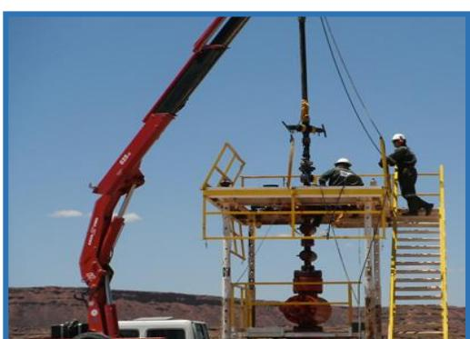
Wireline operations can be done inside the tubing without killing the well, by means of a lubricator connected to the wellhead. Operations can be carried out under pressure and even without stopping production. Further, wireline operations are performed quickly due to the use of lightweight, highly mobile equipment and run by two or three specialized operators. As a result, wireline operations can be readily implemented at relatively low cost.
