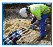
This practical and highly-interactive course includes practical sessions and exercises where participants carryout HV/MV cable jointing, termination, splicing and testing. Theory learnt in the class will be applied using the latest heat-shrink jointing and termination methods suitable for in-class training.
