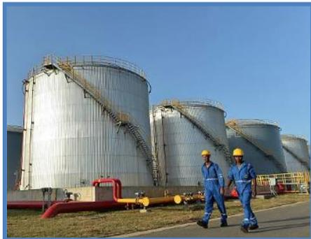
A tank maintenance and integrity evaluation programme can only be effective if it also considers tank design requirements. Recognizing the primary features of these tanks and understanding how they are designed provide the information needed to better understand their maintenance requirements. The course focuses on atmospheric storage tank design requirements in accordance with API 650.
