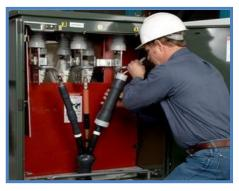
This practical and highly-interactive course includes practical sessions and exercises where participants carryout HV/MV cable jointing, termination, splicing and testing. Theory learnt in the class will be applied using the latest heat-shrink jointing and termination methods suitable for in-class training.
