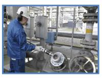
Motor Operated Valve (MOV) is an important item of plant & piping system. These valves are generally of large size and are used for different applications such as pump discharge etc. motor operated valves serve the purpose of fully opening or fully closing valves in pipelines. For example, cooling water lines, process pipelines where controlling of fluid is not required, motor operated valves can be used to fully allow or fully stop the fluid flow.
