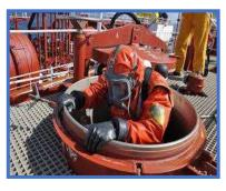
Confined Space Entry (CSE) procedures are made for the safety of those working in confined space. They are designed to prevent accidents and injuries caused by the accidental release of energy. The use of these procedures prevents workers from accidentally being exposed to injurious and even life-threatening situations with energized machinery and equipment.
