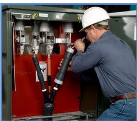
Cable terminations and joints form the weakest link in any distribution system. Also, a failed joint in an underground distribution system is much more difficult to locate and repair compared to any similar problem in overhead distribution systems. This means that we should do our utmost to achieve a good joint or termination, which can give years of trouble-free service.
