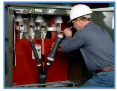
Cable terminations and joints form the weakest link in any distribution system. Also, a failed joint in an underground distribution system is much more difficult to locate and repair compared to any similar problem in overhead distribution systems. This means that we should do our utmost to achieve a good joint or termination, which can give years of trouble-free service.
