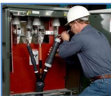
Cable terminations and joints form the weakest link in any distribution system. Also, a failed joint in an underground distribution system is much more difficult to locate and repair compared to any similar problem in overhead distribution systems. This means that we should do our utmost to achieve a good joint or termination, which can give years of trouble-free service.
